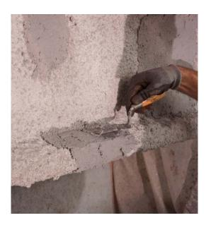
There is a one inch maximum thickness that can be applied in a single pass. Anything above one inch requires multiple coats. Allow material to become stiff but not completely dry before applying the next coat.
