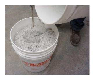
Step 4 – Mechanically mix material for 1-3 minutes until the mix is a lump-free. Hand-held Mixers such as a drill mounted mixer are suitable.
