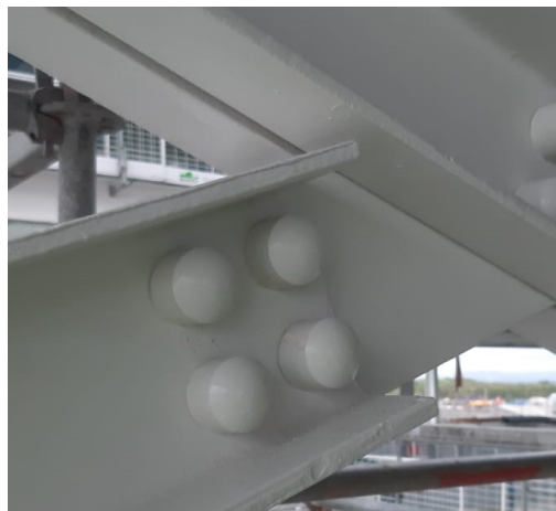
Figure 6. Properly installed bolt caps
