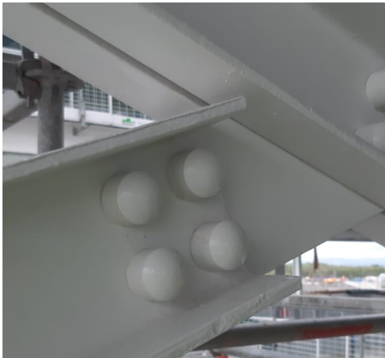
Figure 3. Installed bolted connections.
