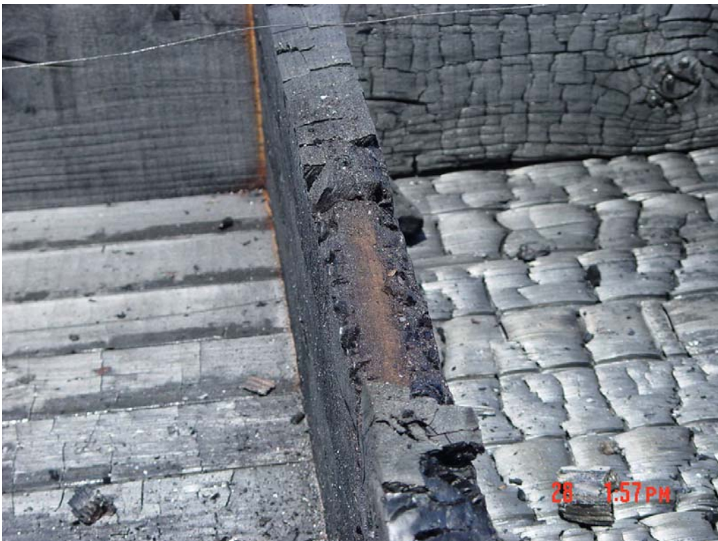
Photograph 12: Close-up of exposed joist with char scraped away
